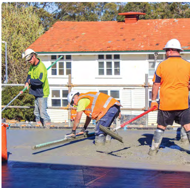
ABOVE: The auditorium is taking shape quickly—the building of the second level has commenced. BELOW: Workers pouring the slab for the second level.
